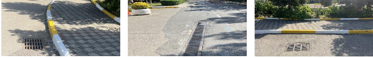
Figure 13. Rainwater gratings
